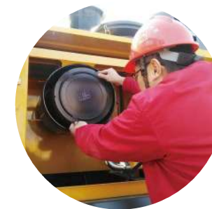
Replace air filter element
